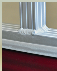
Welded then Anodized Rail Supports
